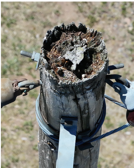
Left: Drone technology provides detailed views of poles and equipment, allowing CVEC to spot a deteriorated pole and make informed maintenance decisions. Right: A CVEC drone inspects electric infrastructure from above.
